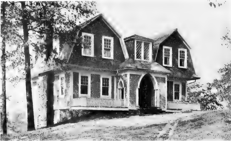
5—This House is Unique in Type, Built of Stone, Stucco and Shingles
